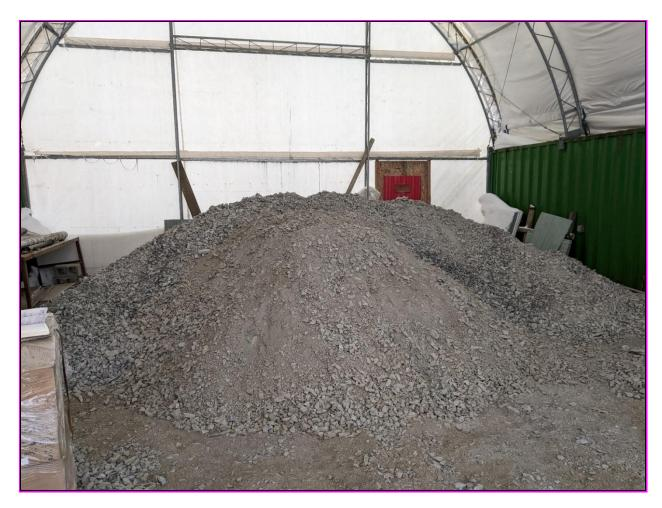
Figure 9-9 Bulk Material stored in a Shelter
