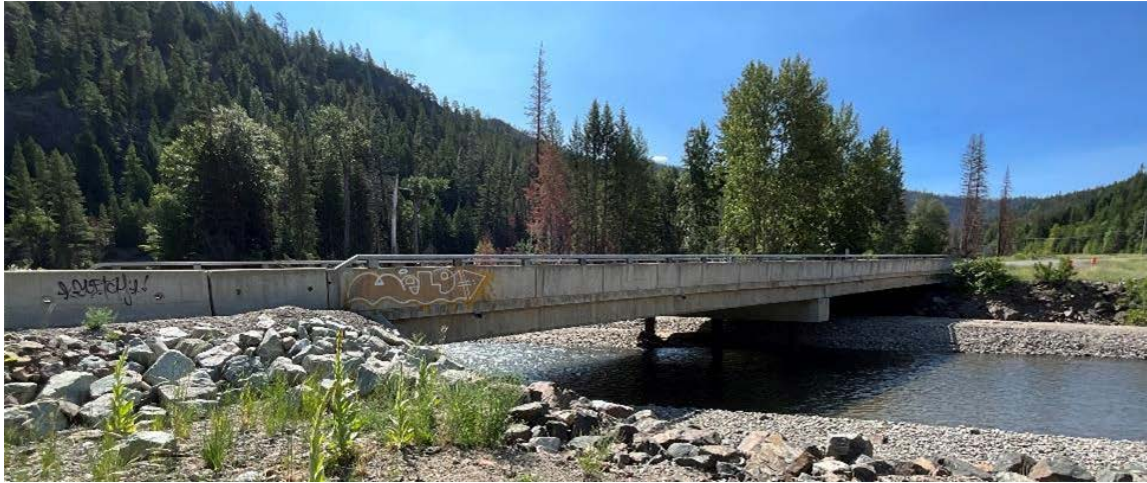
FIGURE 5.5 BRIDGE NO.1 ON THE COLDWATER ROAD
