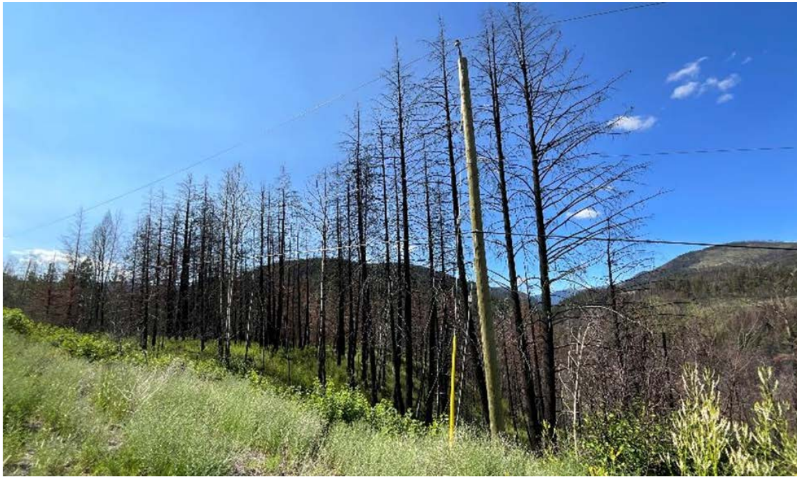
FIGURE 5.7 POWERLINE ALONG THE COLDWATER ROAD
