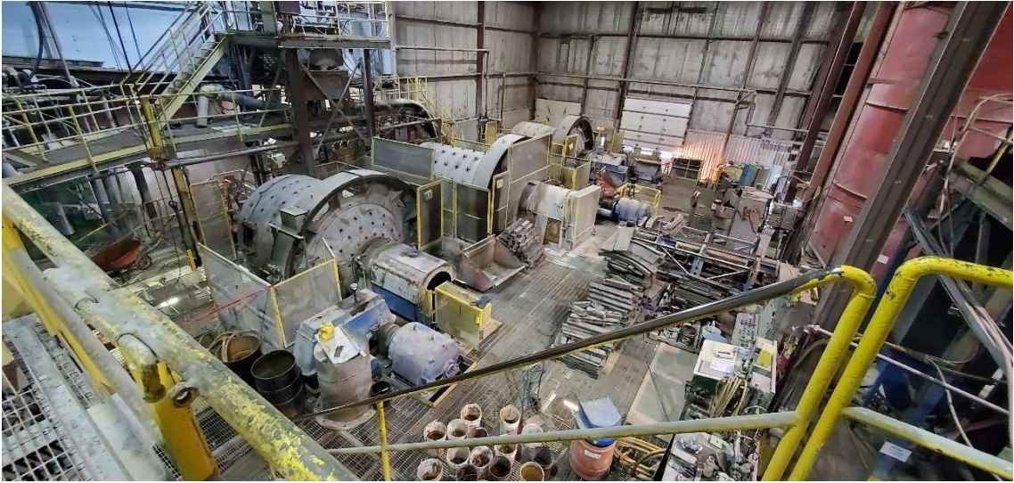
Figure 12.5 – Mill under maintenance (2)
